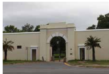
DROSTDY ARCH (SOMERSET STREET)
